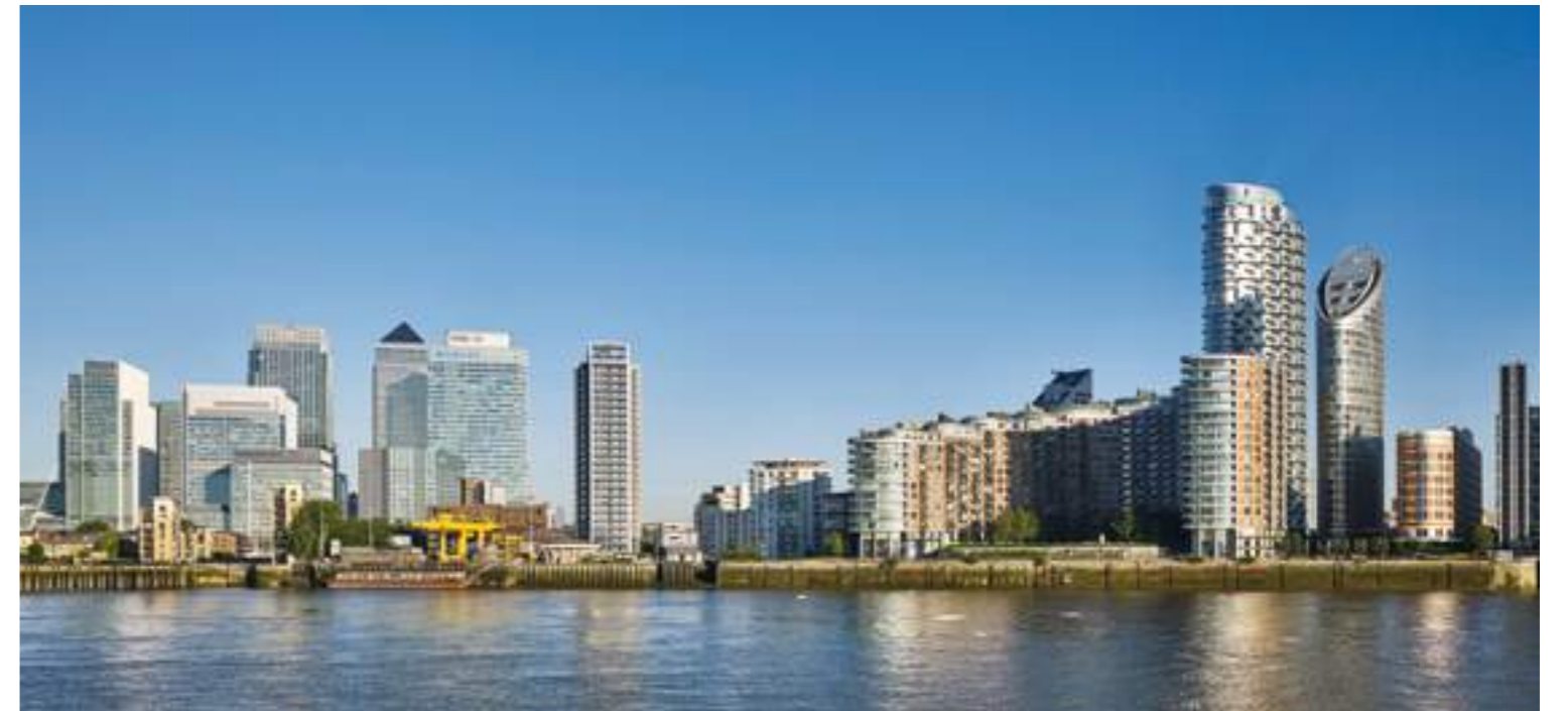
NEW PROVIDENCE WHARF
