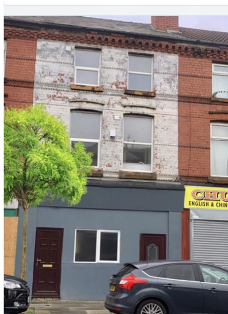
PRIOR TO RENOVATION
